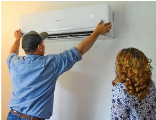
Festus Rockensock shows Bernadette how to keep her mini-split heat pump operating efficiently by cleaning the air filters.
