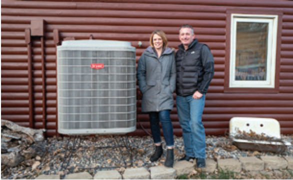
In the winter, cold-climate heat pumps (CCHP) absorb and transfer heat inside, and in the summer the units work in reverse, removing heat from the home.
