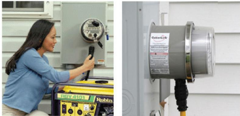
GenerLink™ makes connecting your portable generator easy and safe while providing you the flexibility and control to select what you want to run using your home's circuit panel.
