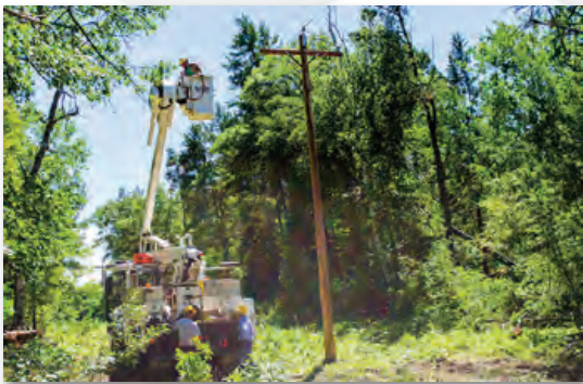
Right-of-way clearing ensures there is sufficient room for maintenance equipment and crews to access and work safely on lines.
